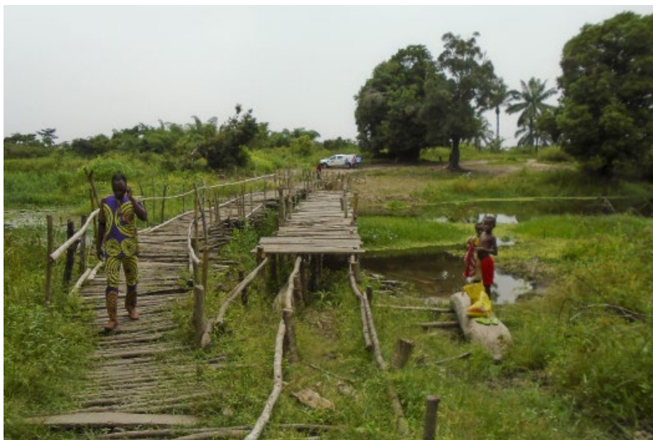
In rural areas, physical access is characterised by footpaths and broken or absent bridges. BENIN
