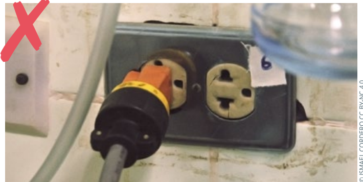
Figure 5 Do not overload electrical outlets by plugging in devices that, together, will exceed the circuit's current limit.
