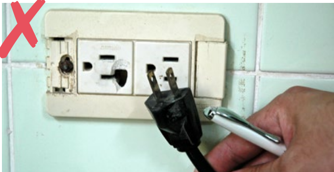
Figure 3 A plug with the ground wire pulled out, which is very dangerous. Do not use.
