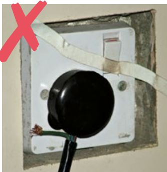
Figure 3 A plug with the ground wire pulled out, which is very dangerous. Do not use.
