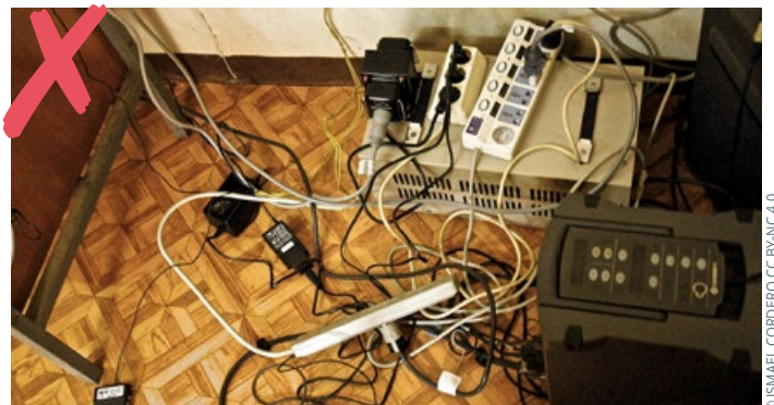
Figure 5 Do not overload electrical outlets by plugging in devices that, together, will exceed the circuit's current limit.
