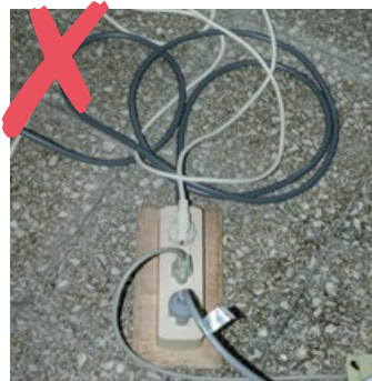
Figure 4 Do not run cords along the floor, as they may cause a tripping hazard.
