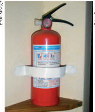
Dry powder fire extinguisher. Note the white pointer on the dial is in the green (safe) range. Check it annually with the fire department.
